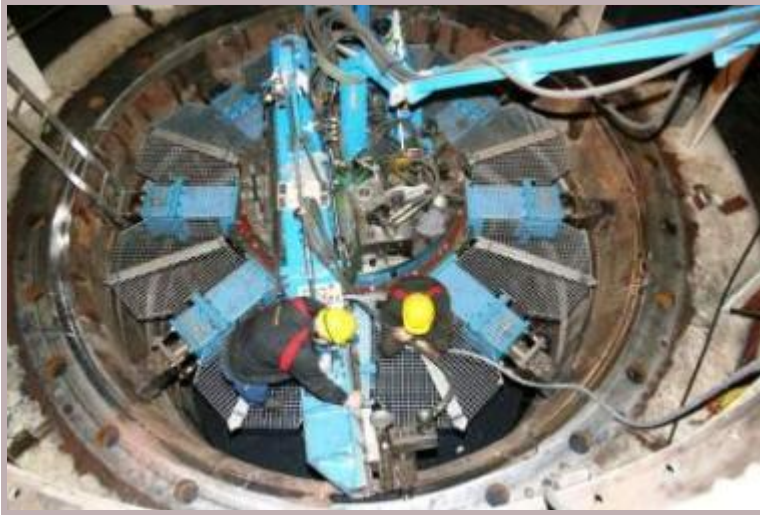
Special machine-tools for on-site machining
